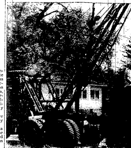
It took quite a bit of sidewalk supervision as well as work by both men and equipment to remove this large stump from the lot on which the new REA building is being constructed. A Watson Brothers crane truck from Omaha was needed to lift the stump and place it on the truck for hauling away. Frank Thielman is supervising construction of the new building.
